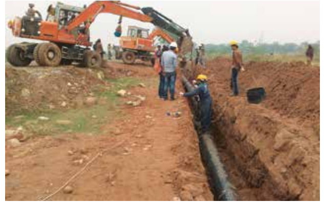
The Soda Ash project team laid a new water pipeline using steel mesh reinforced polyethylene pipe.
